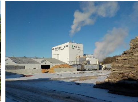
Kobe Bussan's Woody Biomass Power Plant
