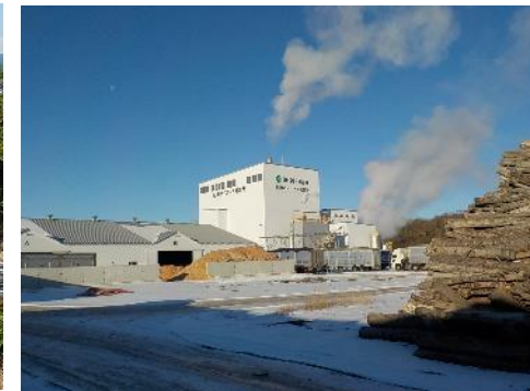
Kobe Bussan's Woody Biomass Power Plant
