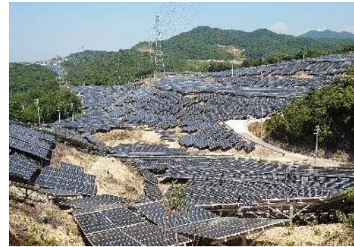
Kobe Bussan's Solar Power Plant (Photo: The plant in Misaki-cho generates 9.9 MW.)
