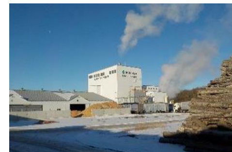
Kobe Bussan's Woody Biomass Power Plant
